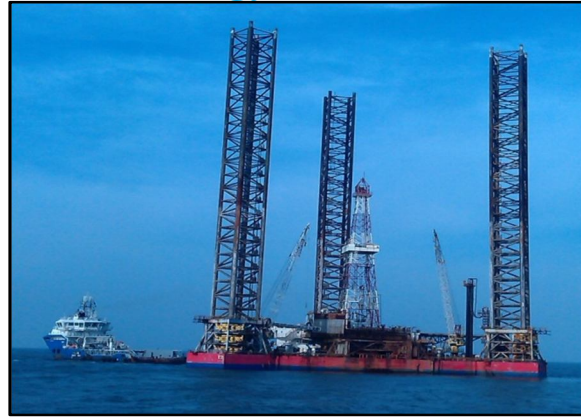
Fig-2: Rig with legs elevated and floating condition
