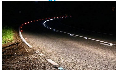
Figure 1: Illuminated solar road [1]
