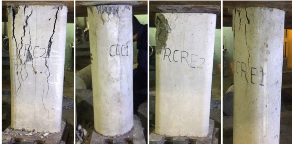
Fig. 9: Failure of Control Specimen and FECC
