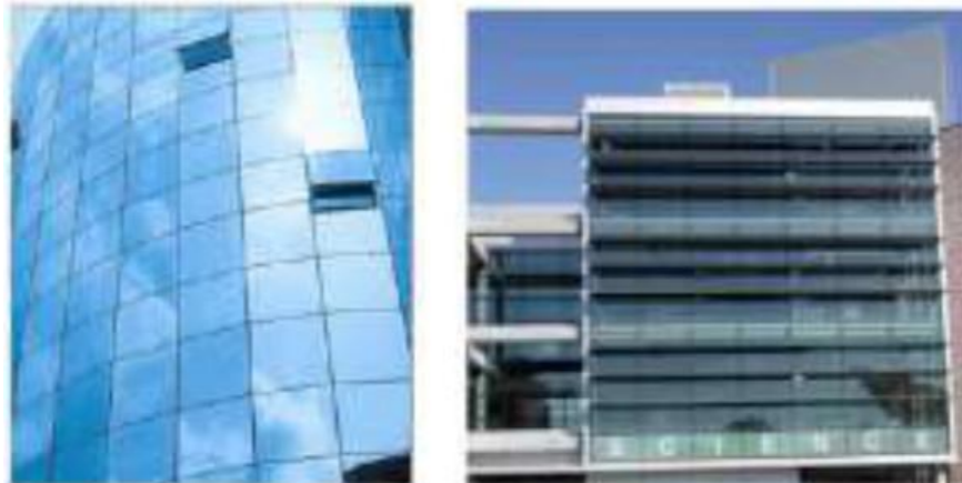
Fig.7. SCFW Glazing System Implemented in a Building at tiruchirapalli district.
