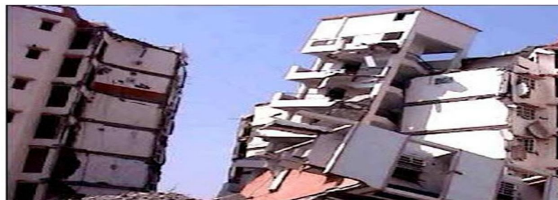
Fig. 2:- Collapse of a Building
