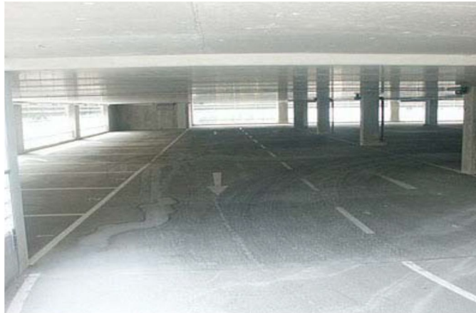
J. Car park built with Bubble Deck in Frankfurt, Germany
