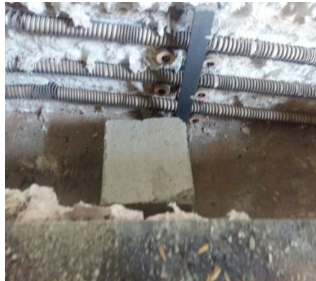
Fig.5 Fire Resistance Test
