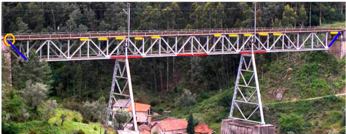
Fig. 7: Fatigue critical locations.
