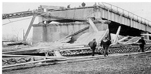
Fig.1 : Silver Bridge Failure
