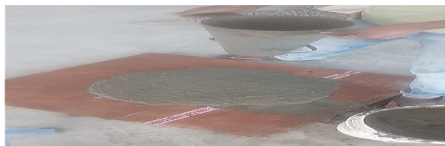
Slump Test for SCC
