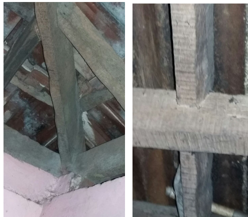
Fig. 8 Wall plate and rafter-purlin joinery
