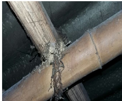
Fig. 10 Joinery using coir
