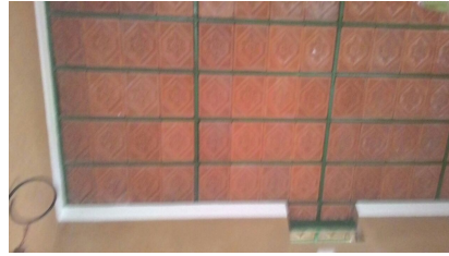
Fig. 3 Mangalore tiles laid exposed to the interior.
