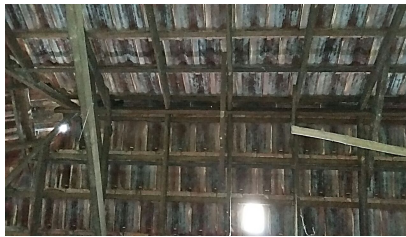
Fig. 7 Tiled roofing on coconut-framed structure
