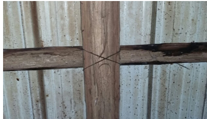
Fig. 11 Joinery using metallic threads-areca framed structure
