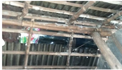
Fig. 9 Sheet roofing on bamboo-areca framed structure
