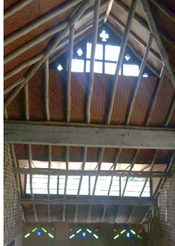
Fig. 5 Bamboo ply on Casuarina framework and gable windows promoting ventilation
