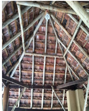
Fig. 6 Tiled roofing on Casuarina framed structure
