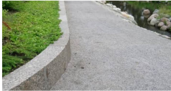
Fig.1 Stone dust used for yard construction
