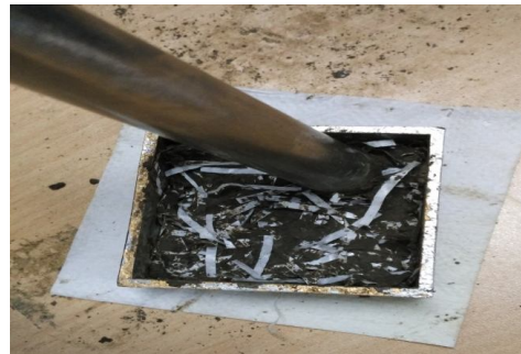
Figure 3.2 compaction of material
