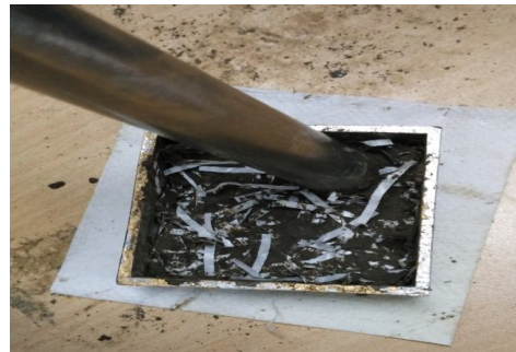
Figure 3.2 compaction of material
