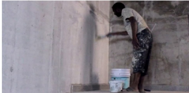
Figure 10 Painting and finishing works
