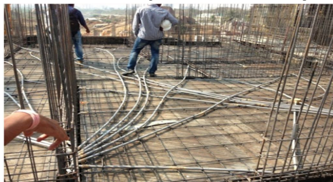
Figure 5. Horizontal reinforcement of shear wall
