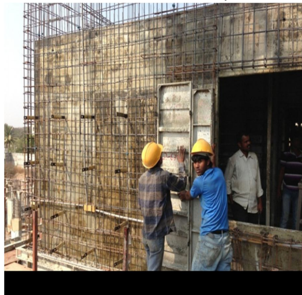
Figure 7. MIVAN formwork
