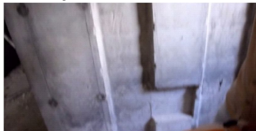
Figure 5 Gaps left for plumbing lines
