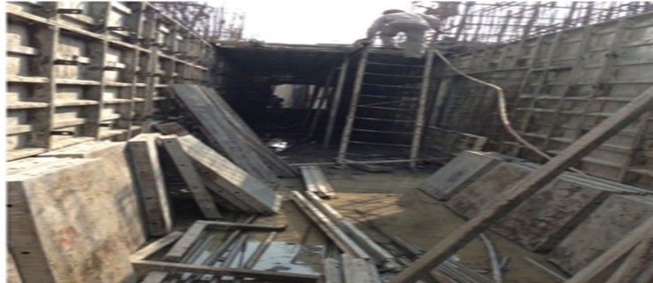
Figure 2 Alluminium panels of MIVAN formwork
