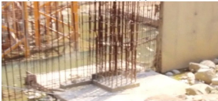
Figure 4. Footings laid for construction
