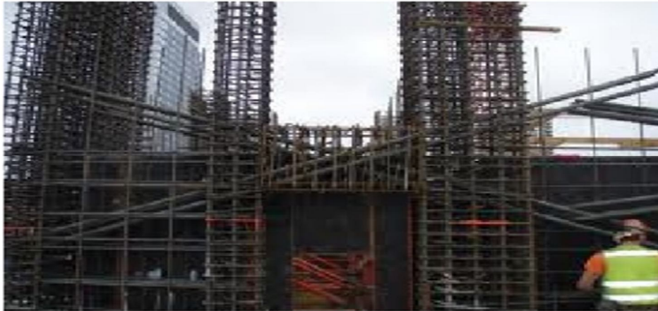
Figure 1 R.C Shear wall
