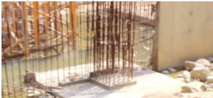
Figure 4. Footings laid for construction
