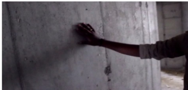
Figure 6 Shear wall after removal of formwork
