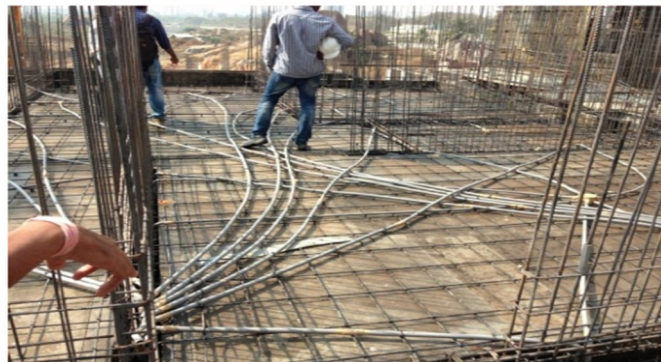
Figure 5. Horizontal reinforcement of shear wall
