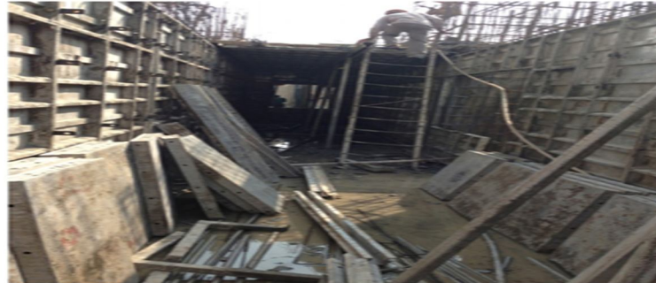
Figure 2 Alluminium panels of MIVAN formwork
