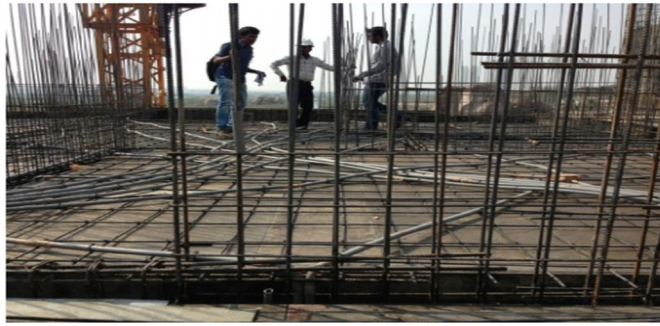
Figure 6. Vertical Reinforcement of shear wall
