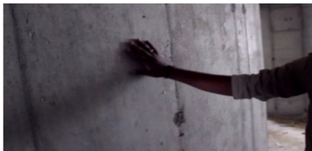
Figure 6 Shear wall after removal of formwork
