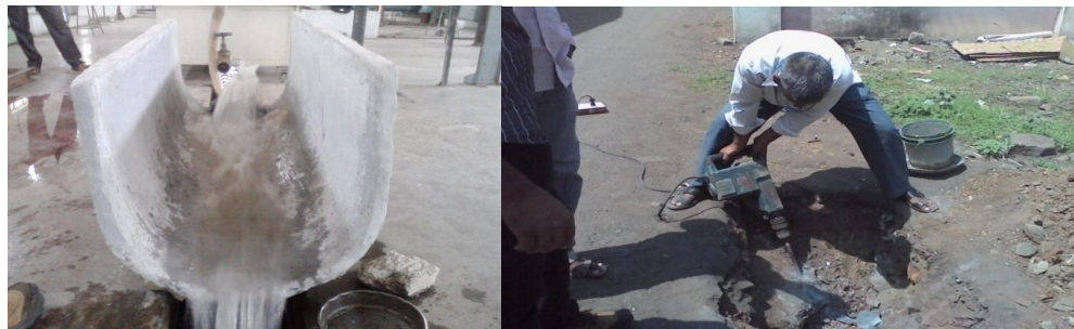
PHOTO 3.18 – Scouring test & excavation
