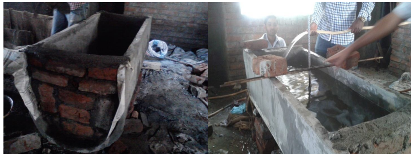
Photo 3.9 - Bund construction & Setup for leakage test.
