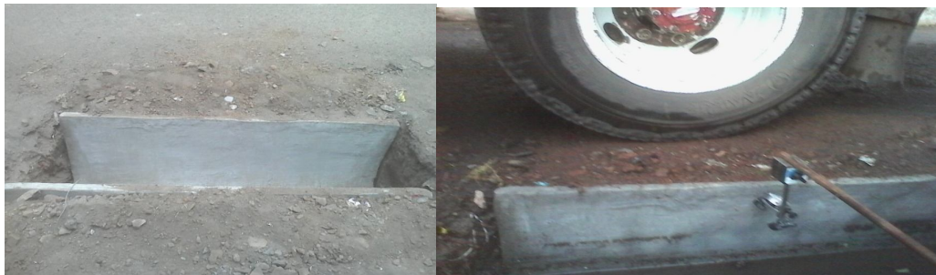
PHOTO 3.20 – Placing of gutter & Deflection test.
