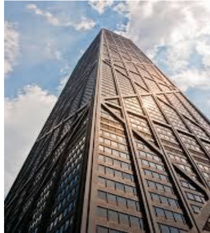
Fig.1 Braced tube structure (John Hancock Center)
