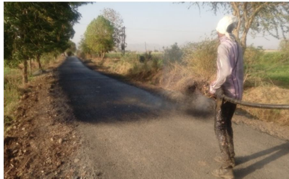
Fig-4 Bituminous mix lying on site
