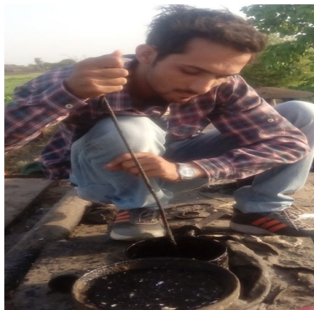
Fig - 4: Stirring of added waste plastic in bowser
