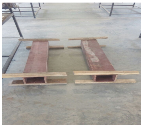
Figure 3: Special Timber Formwork
