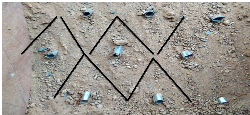
Fig.11 Staggered or Triangular Nail Pattern
