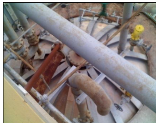
Fig. 4 Radar Location "Hopper Worn FC-D-509".
