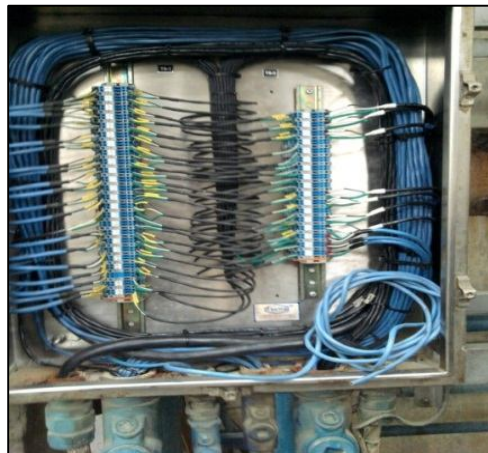
Fig. 7 Interior Junction Box Terminal.
