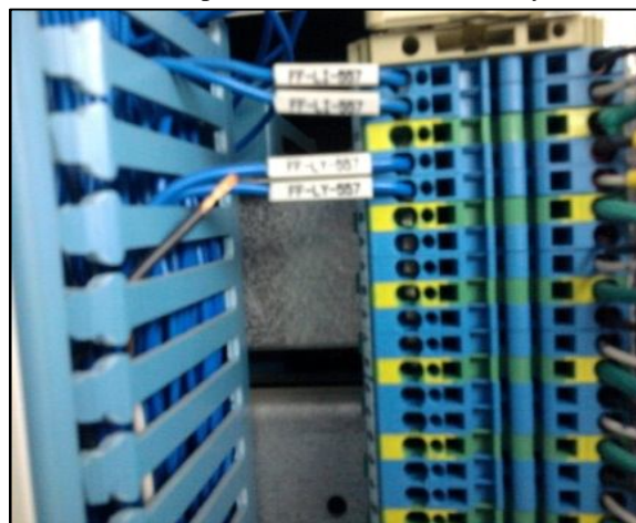
Fig. 11 Terminal block. Arrival of Radar Threads
