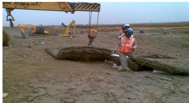
Laying of blasting pads by hydra
