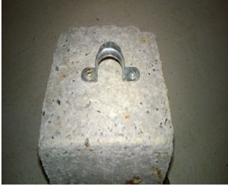
Fig.Channel in the brick
