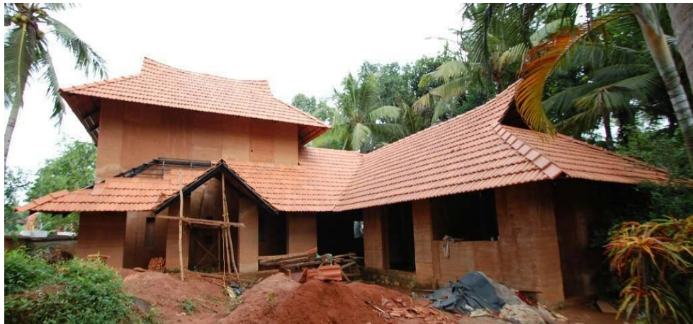
Figure 2: Construction of cement stabilized rammed earth building at Kerala. ( www.inspirationgreen.com )
