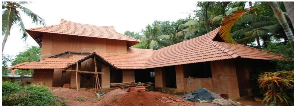
Figure 2 Construction of cement stabilized rammed earth building at Kerala. ( www.inspirationgreen.com )
